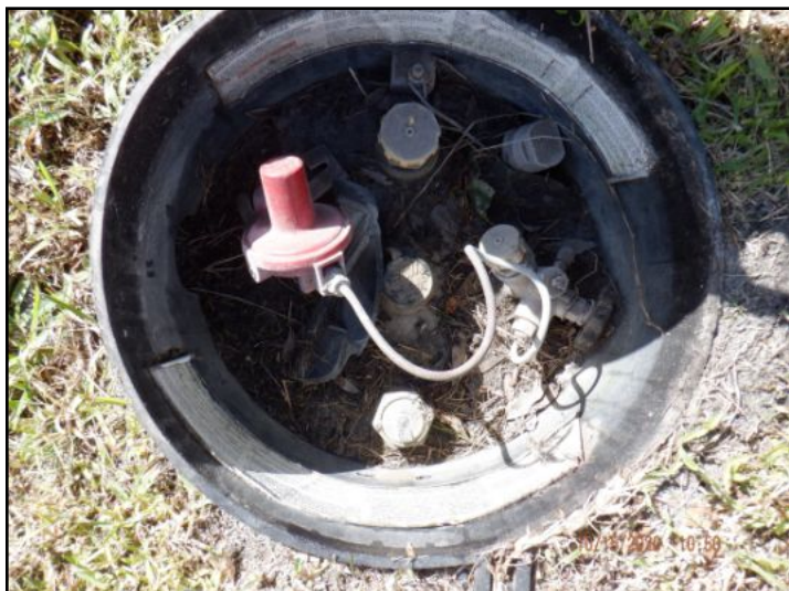
West Tank underground
