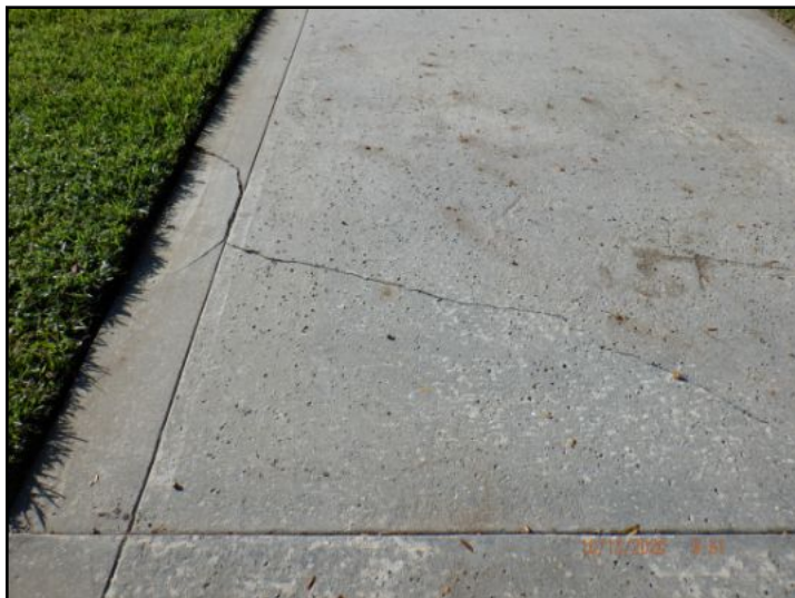
Settlement cracks
