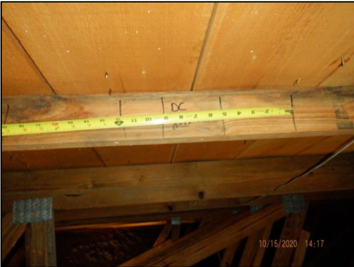
Deck nailing pattern
