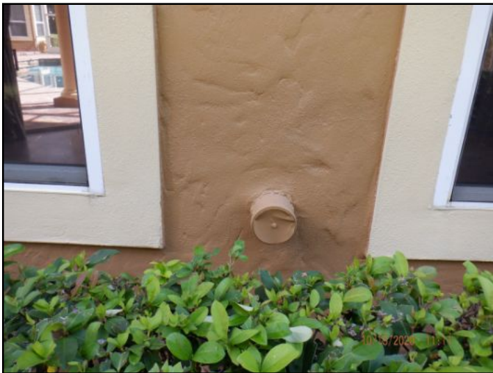
West clean out
