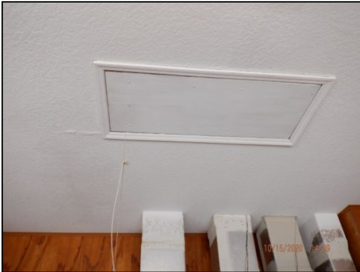
Pull down in garage
