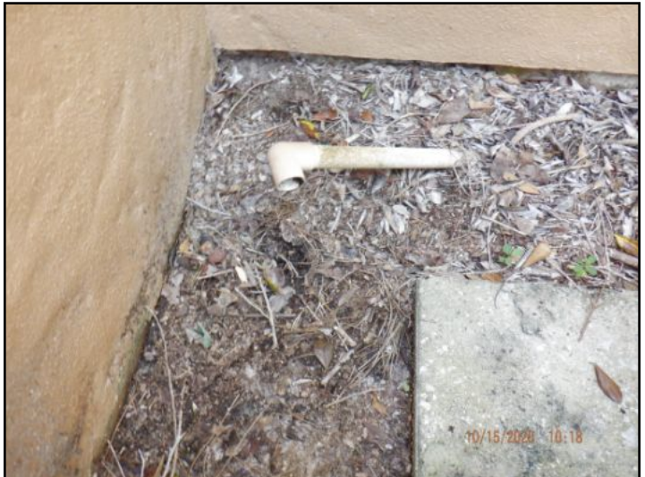
East drain line
