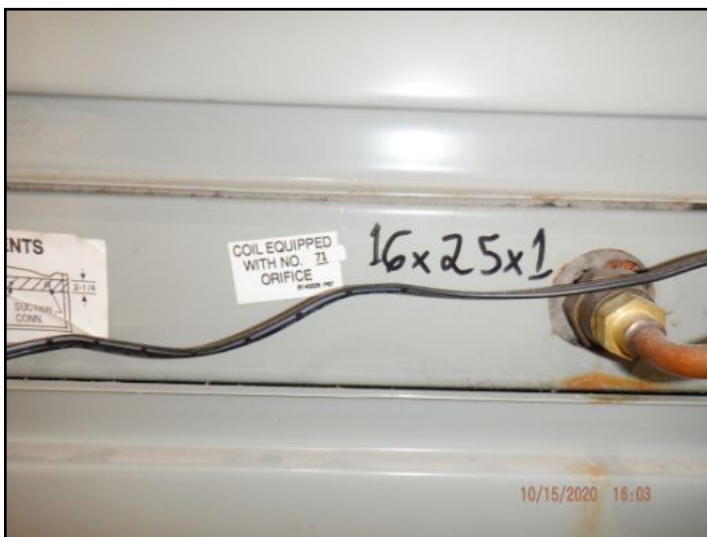
Master air handler filter 16x25x1
