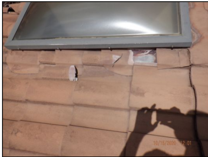
Flashing damage
