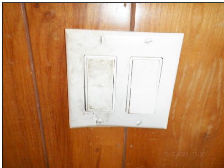
Switch cover damage
