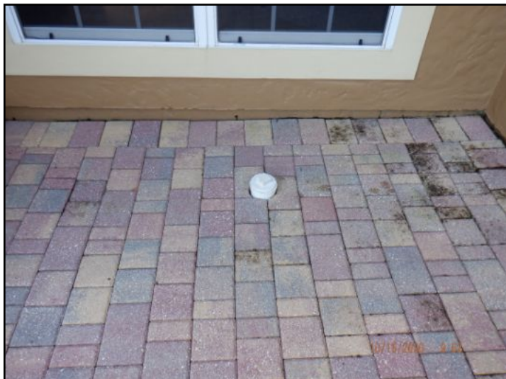
Clean out locantion North exterior
