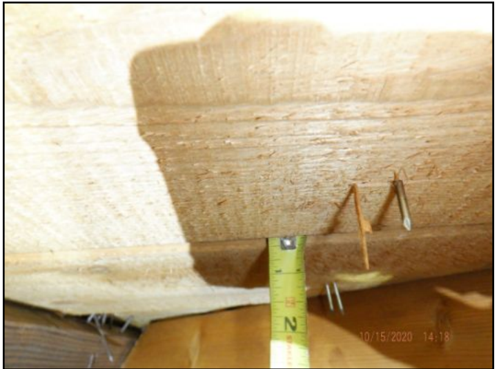
Deck 1/2 inch planks
