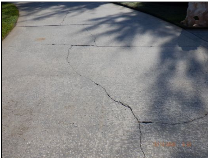
Settlement cracks
