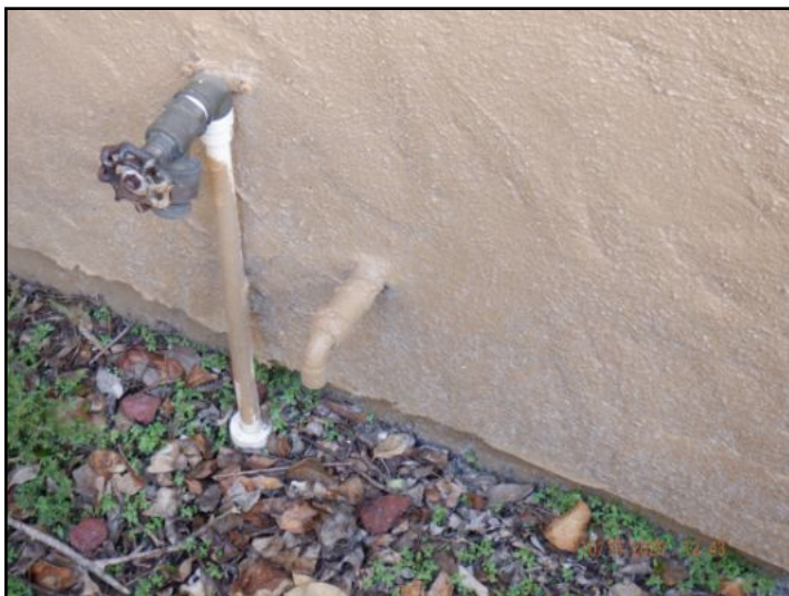
Drains on exterior
