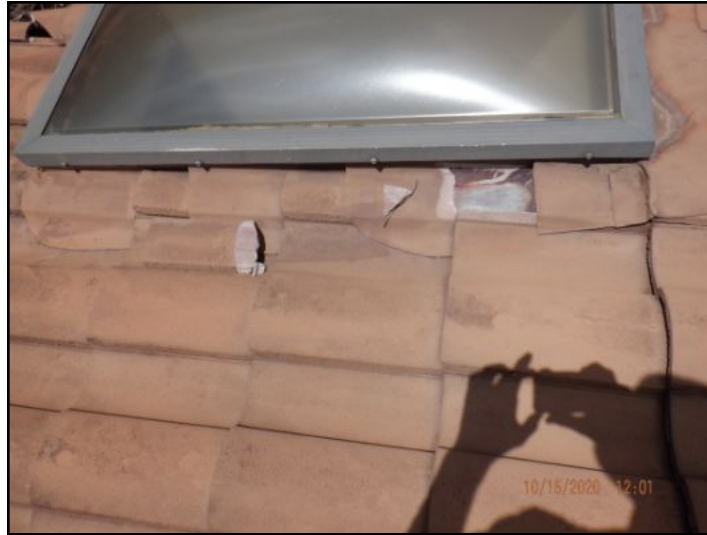
Flashing damage
